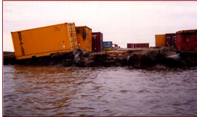
Container storage endangered by Ninglick River erosion.
