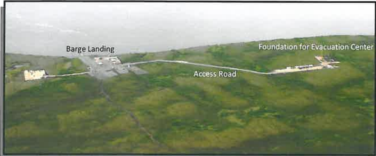
Mertarvik Barge Landing, Access Road & Evacuation Center Foundation. (Harvey Smith, ADOT&PF, 6-2011)
