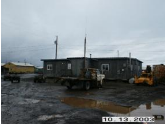
Figure 11: Savoonga IRA hall and office building
