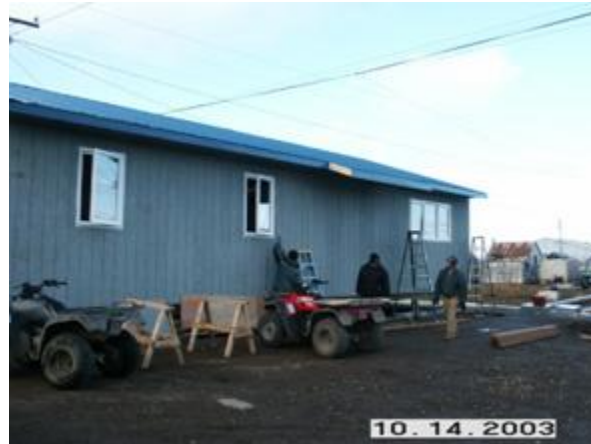
Figure 36: New HIP house in Savoonga being built with local hire crew
