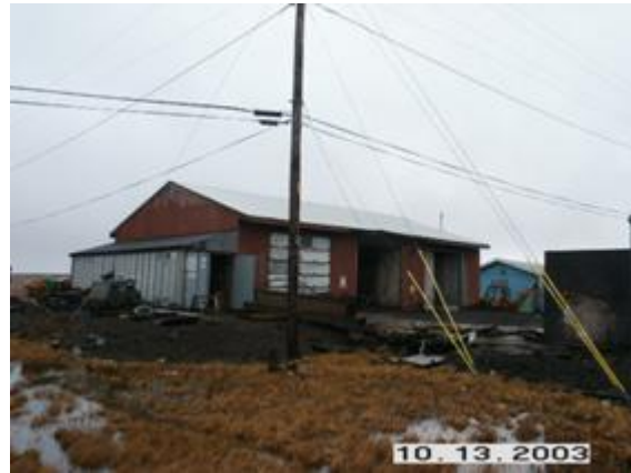
Figure 17: City of Savoonga garage
