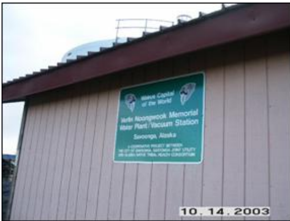
Figure 24: Savoonga water system building
