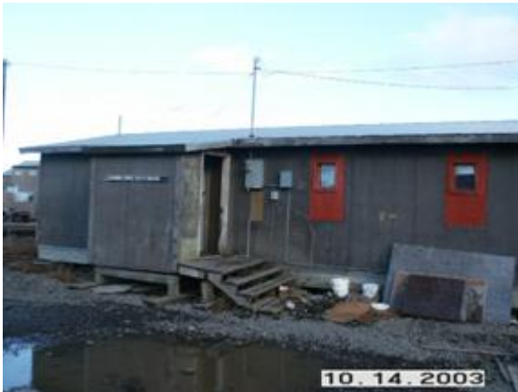
Figure 20: Public Safety building
