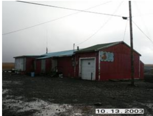
Figure 19: Savoonga fire hall and building
