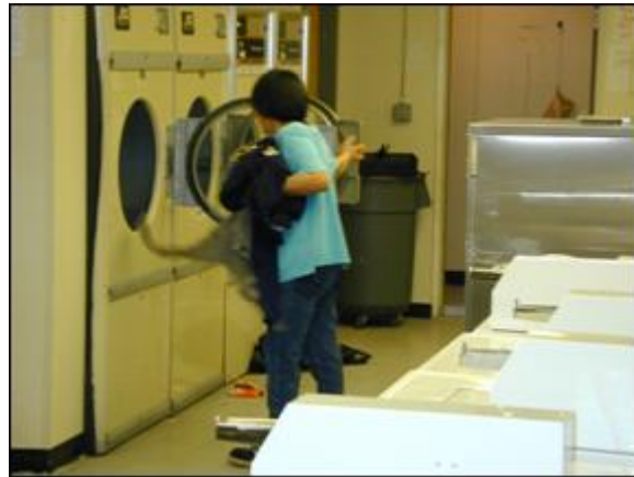
Figure 23: Inside the washeteria
