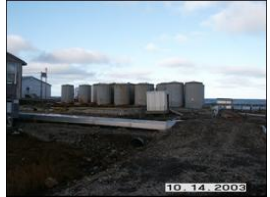
Figure 30: Old School fuel tanks
