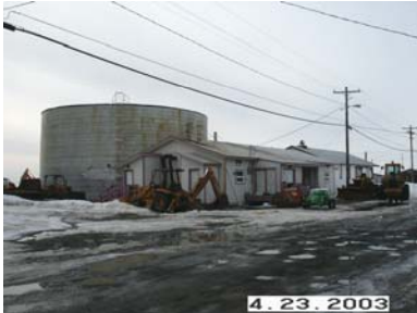
Figure 10: Shaktoolik washeteria and water storage
