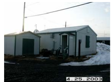
Figure 11: Shaktoolik Tel Alaska building
