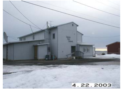
Figure 6: Shaktoolik Native Corporation office building
