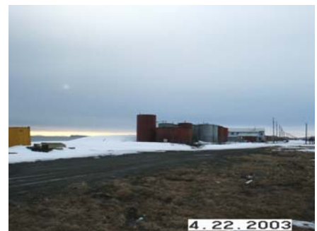
Figure 13: Shaktoolik bulk fuel storage tanks
